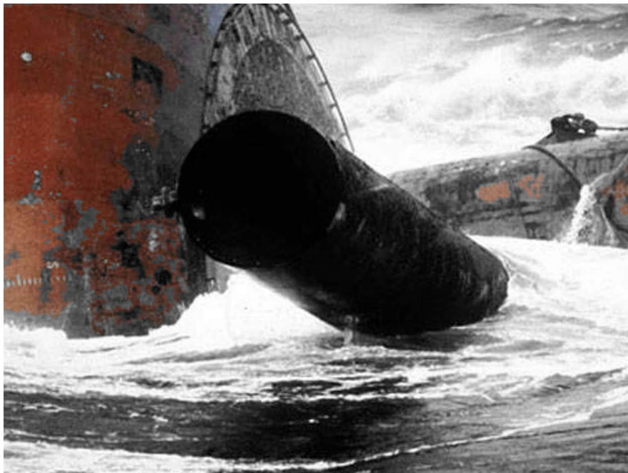
Figure 2 : No evidence of plastic deformation in the product forms e.g. the brace D6, view the back ground of image at the column D and the float chamber, that constituted the platform overall structure, therefore no evidence of overload.
