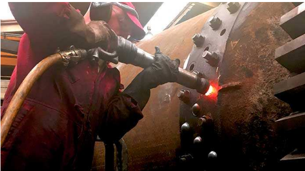
Figure 8. Hot rivet forge welding.
