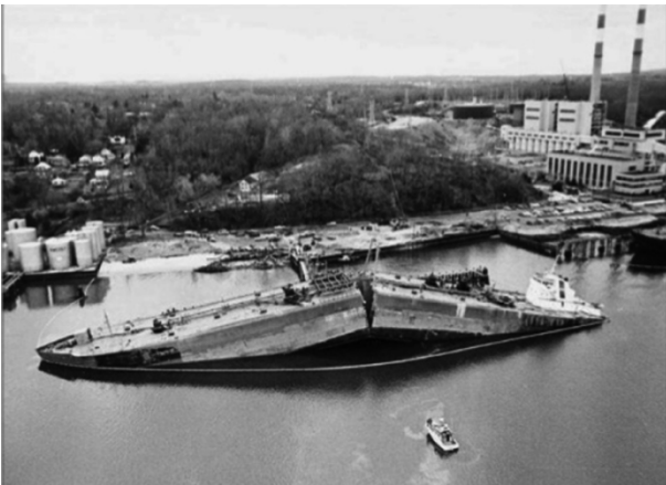
Figure 12. Brittle fracture of a Liberty ship upon launching.
